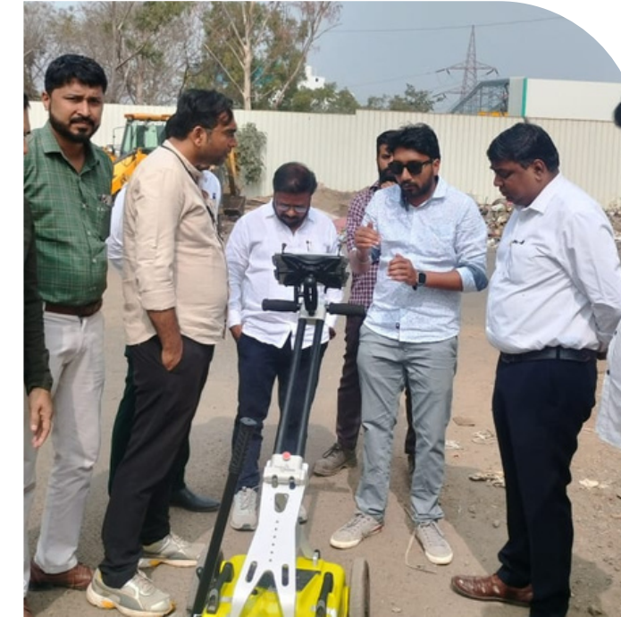
CLIENT: MICROSOFT, CHINCHWAD AGENCY: TEJAS ELECTRICALS DISTANCE: 4KM
